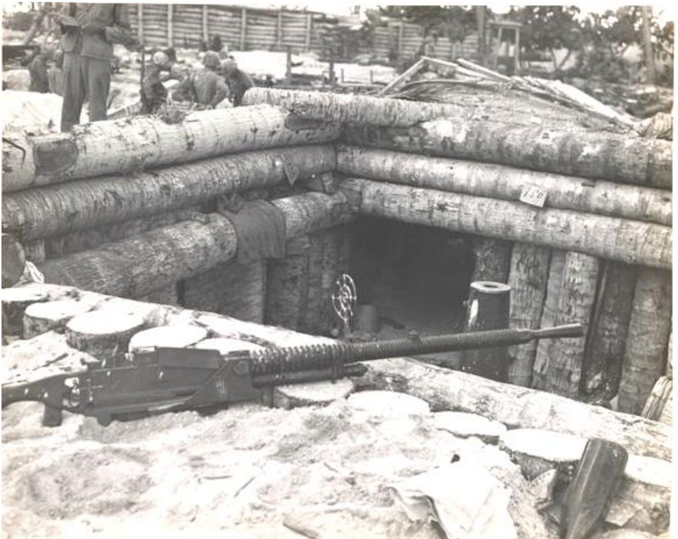
Captured Japanese dugout and communications post
