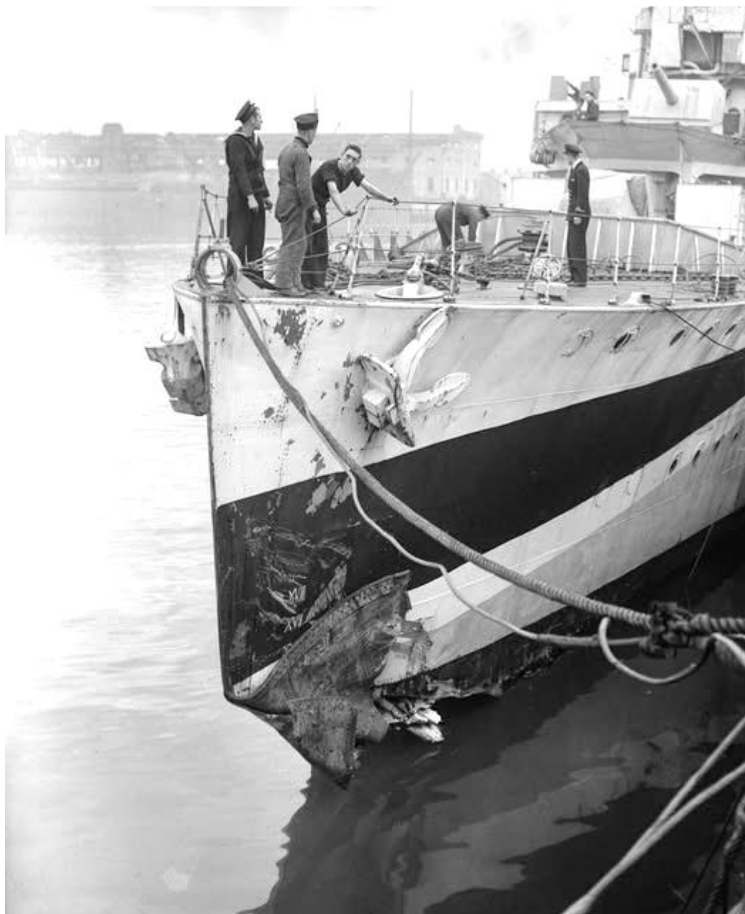
The stem of HMS Viscount, buckled in after ramming a U-boat
