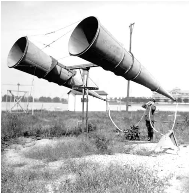
Acoustic locator, 1920s–30s — an early aircraft detection system that relied on sound before radar transformed air defense.
