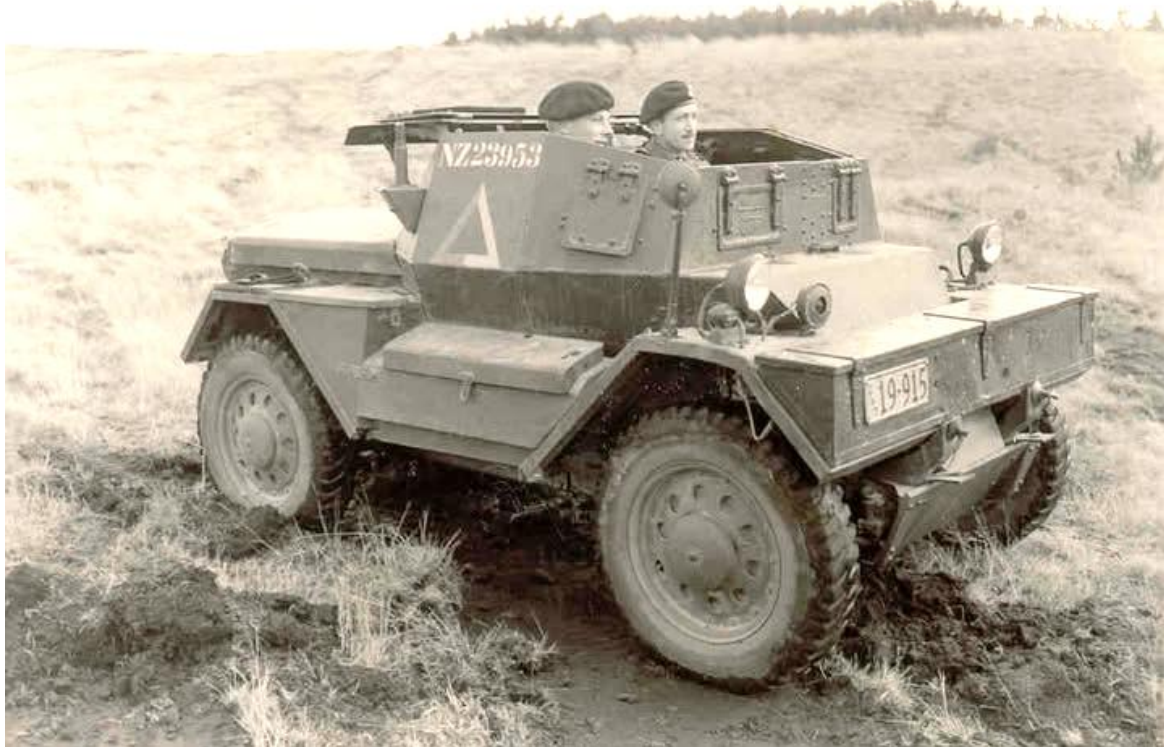
Daimler Dingo NZ23953 in Waiouru note the use of Headlights and sidelights from a Stuart tank
