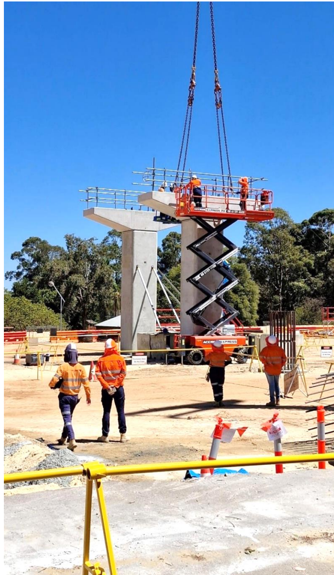
Progress including the headstocks
