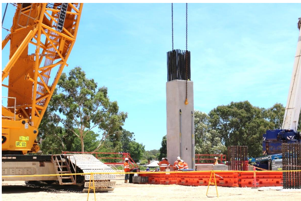
The first column being put into place
