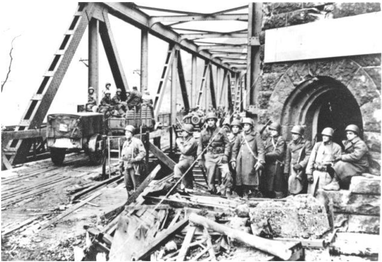
The Ludendorff Bridge between 8 and 11 March 1945
