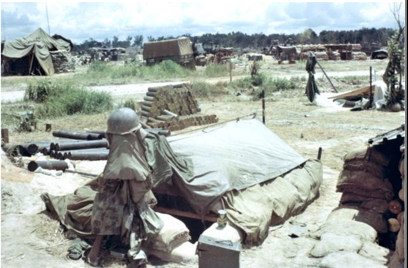
A typical shelter at Coral: the sandbagged cover over the roof offers protection from the weather and, more importantly, from enemy fire. Few, if any, such shelters existed on the first night at Coral, but after the fierce North Vietnamese assault, men were quick to prepare safer pits
