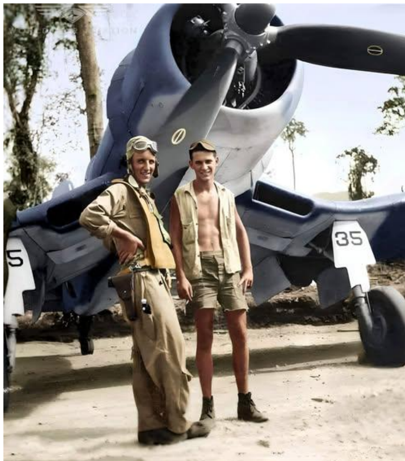
Pilot Hal Bitzegio and a ground crewman by F4U-1A Corsair of the VF-17 Jolly Rogers at Ondongo, New Georgia, November 1943.
