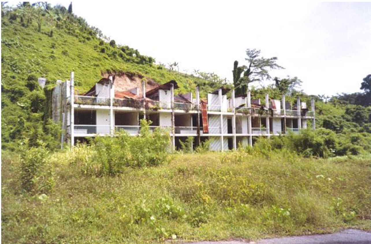
Destroyed resort buildings at Kieta, damaged during the conflict on Bougainville, which lasted for nearly 12 years
