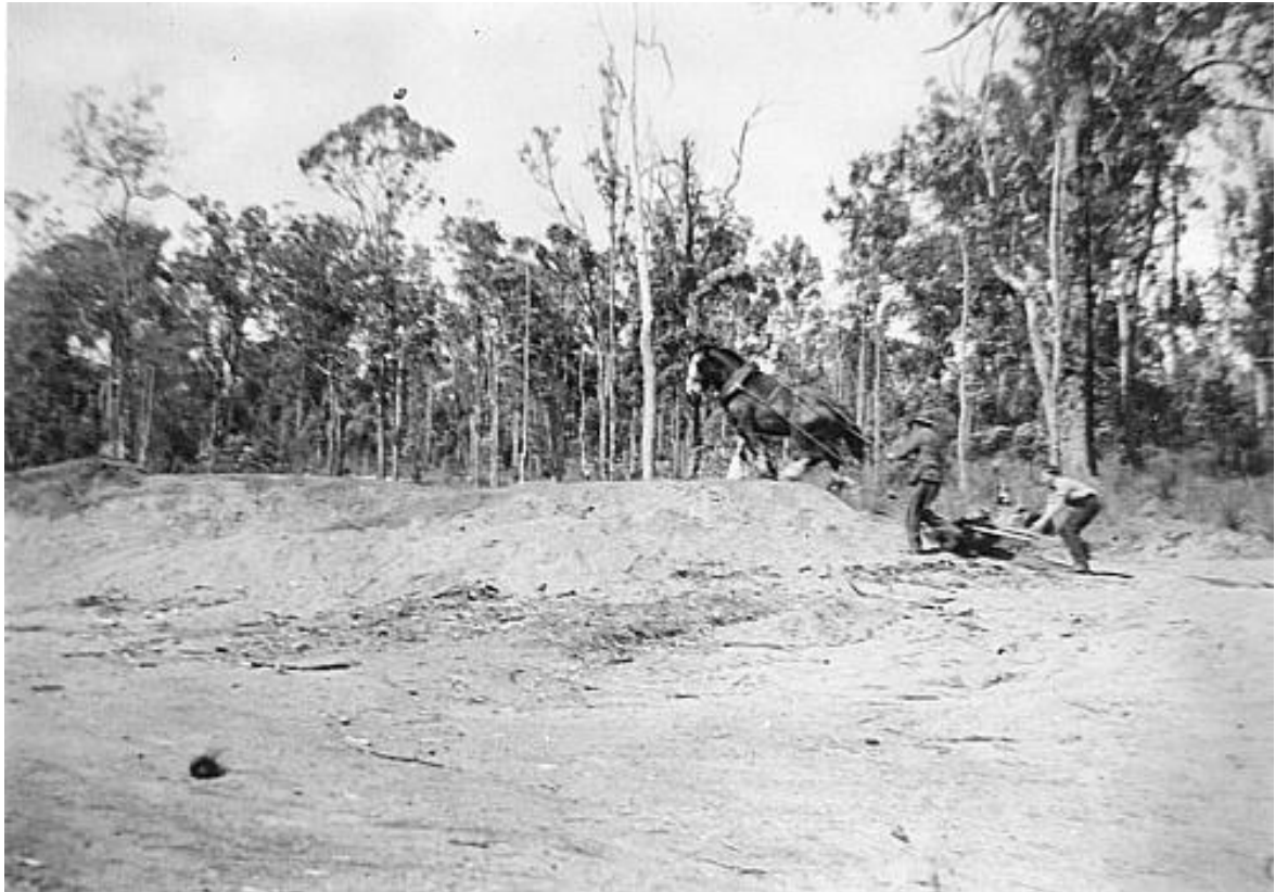
ABOUT TO UNLOAD SCOOPFUL OF SOIL DURING CONSTRUCTION
