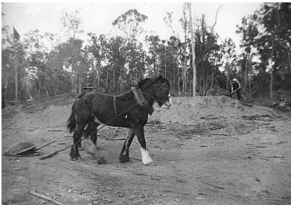
HORSE PULLING A DRAG SCOOP DURING CONSTRUCTION
