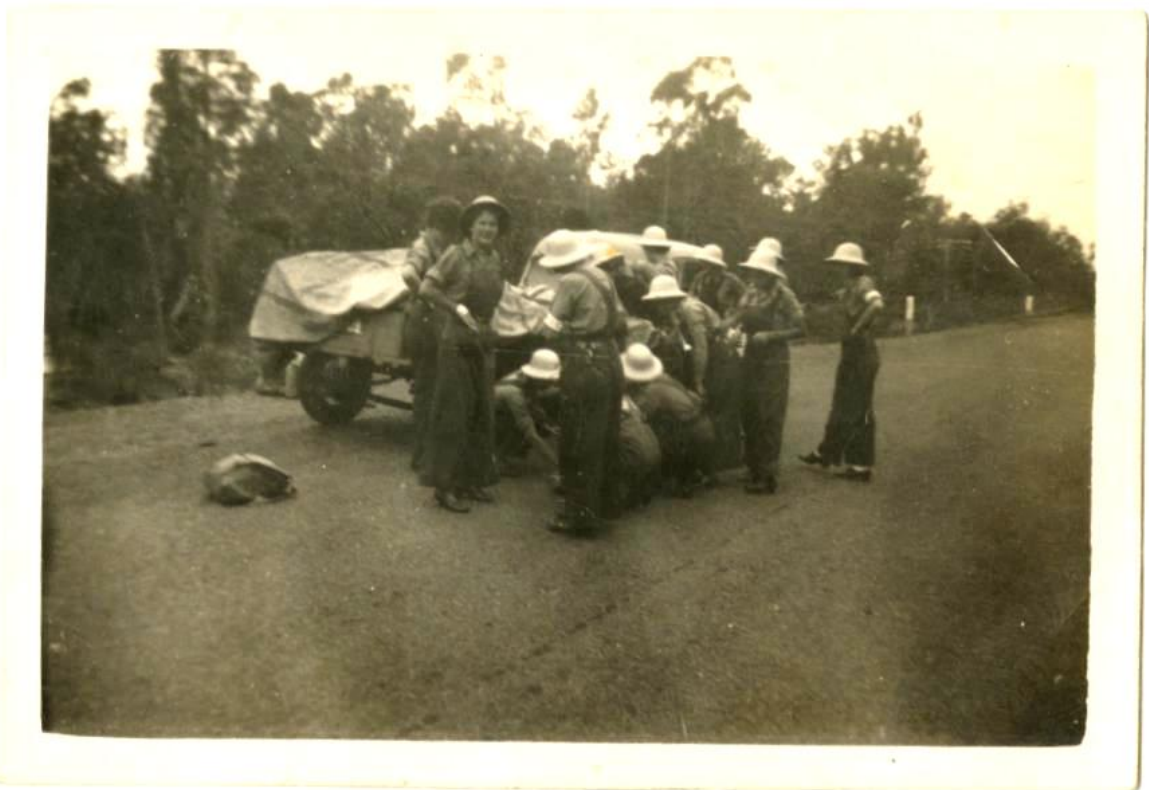
Roadside repairs to trailer en-route to the camping exercise at Turtle Pool, Gleneagle
